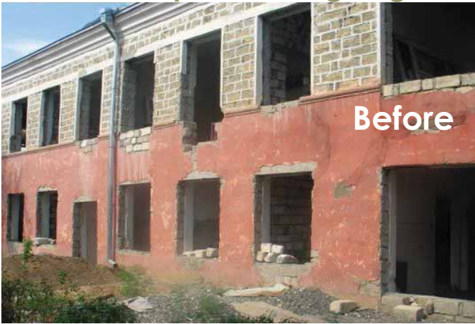
Martuni regional hospital before reconstruction.
