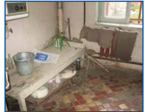
Old Martuni hospital: utility room.
