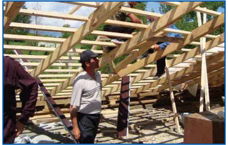
Nearly 500 Shushi residents finally have a safe roof over their heads.
