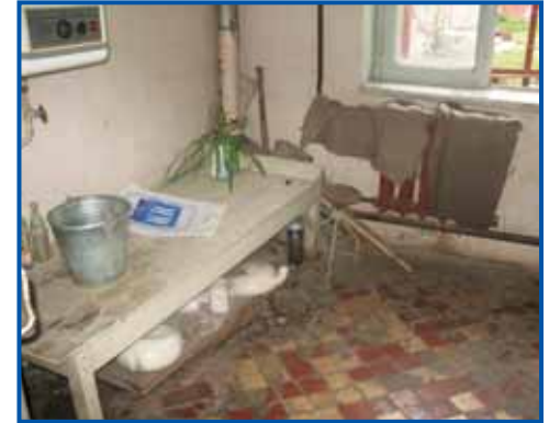
Old Martuni hospital: utility room.
