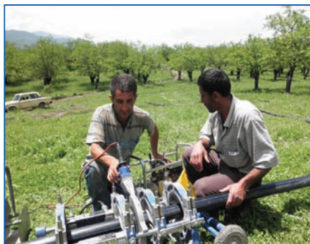
Connecting the pipes that will complete the village's water distribution network.
