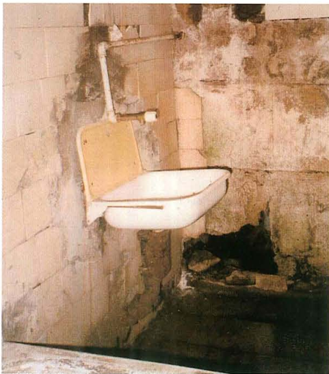
The clinic has no running water and only one toilet.
