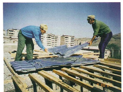
The Vanadzor School is due for completion in the fall of 2001.
